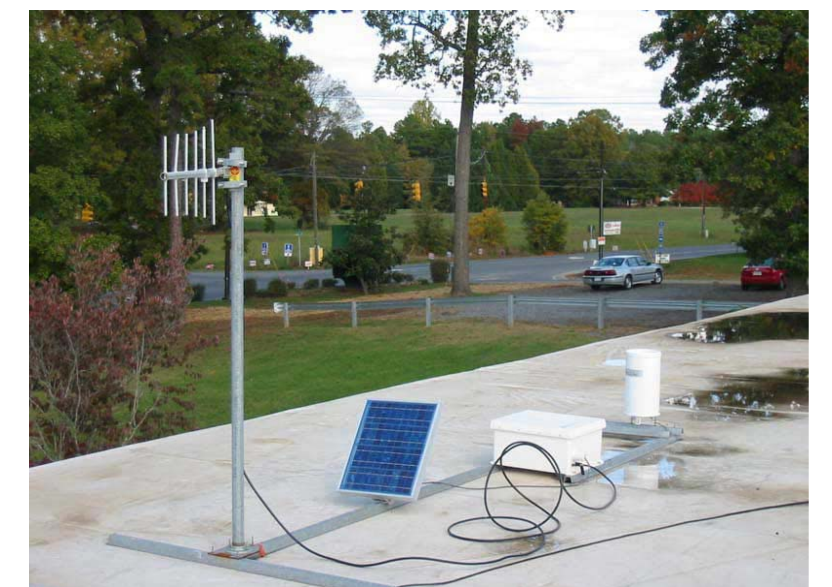
Typical rain gage installation with UHF telemetry atop Odell Elementary School.
